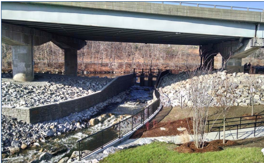
The upper portion of the Tingue Dam fishway (see cover for a photo of the lower portion).
