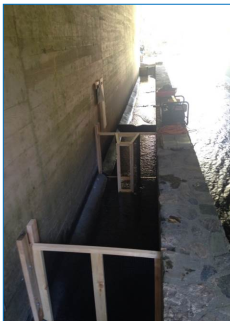
(left) Sun glare hides the lower fishway but the upper fishway (under the culvert) can be seen with the new trap, designed to retain trout for monitoring and fishway evaluation.
