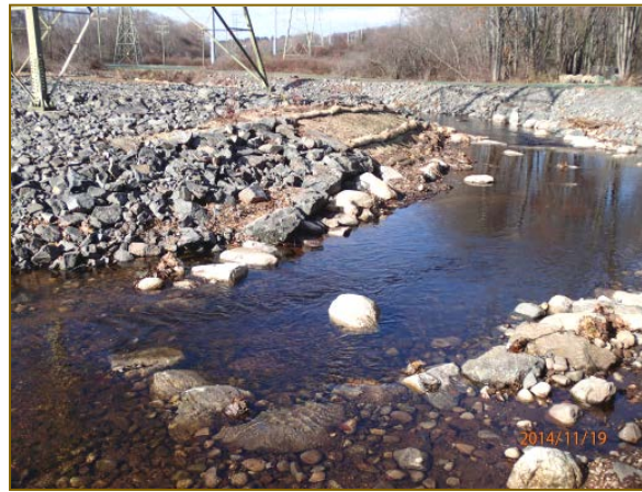
(left) Newly restored Hop Brook stream channel. (right) One of five boulder cross vanes installed in Hop Brook.
